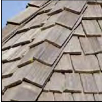
Replicate original wood shingles in exposure, pattern and thickness.
