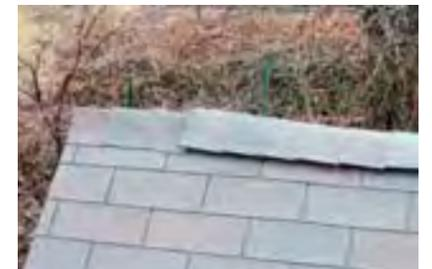
Ridge caps for asphalt shingles should terminate before the eaves, as above, not carry through as below.
