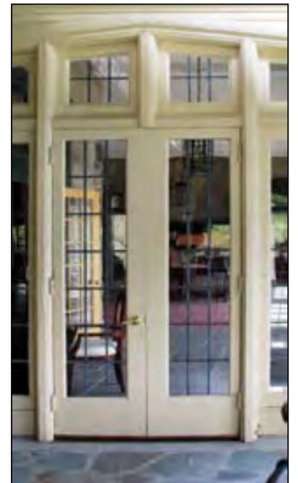
*Repair or replacement of doors with significant glass components should comply with both door and window guidelines.*
