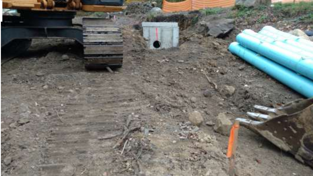
View of Pond No. 3 start of LLO siphon system construction. Photo shows valve vault set to grade near dam crest.
