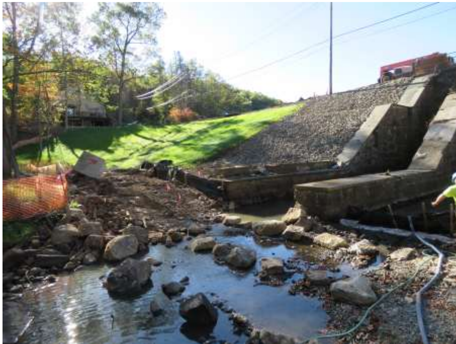
Right Side of Downstream Embankment Slope showing completed rip rap and earth embankment. Seepage collection and monitoring system is not complete along service discharge channel.
