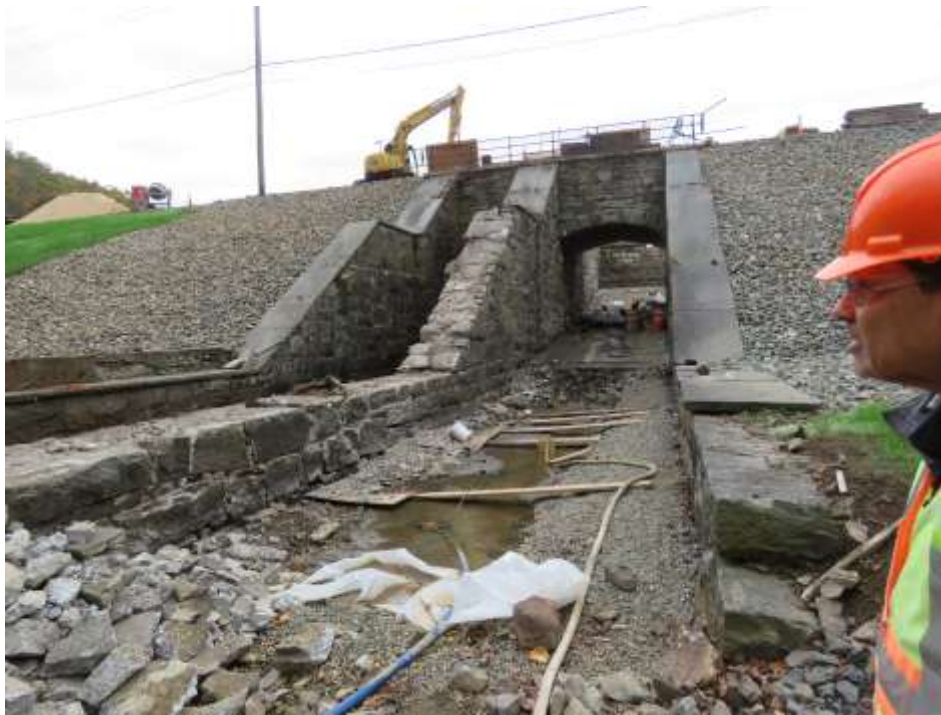
Remove of old concrete “capstone” for installation of new bluestone.
