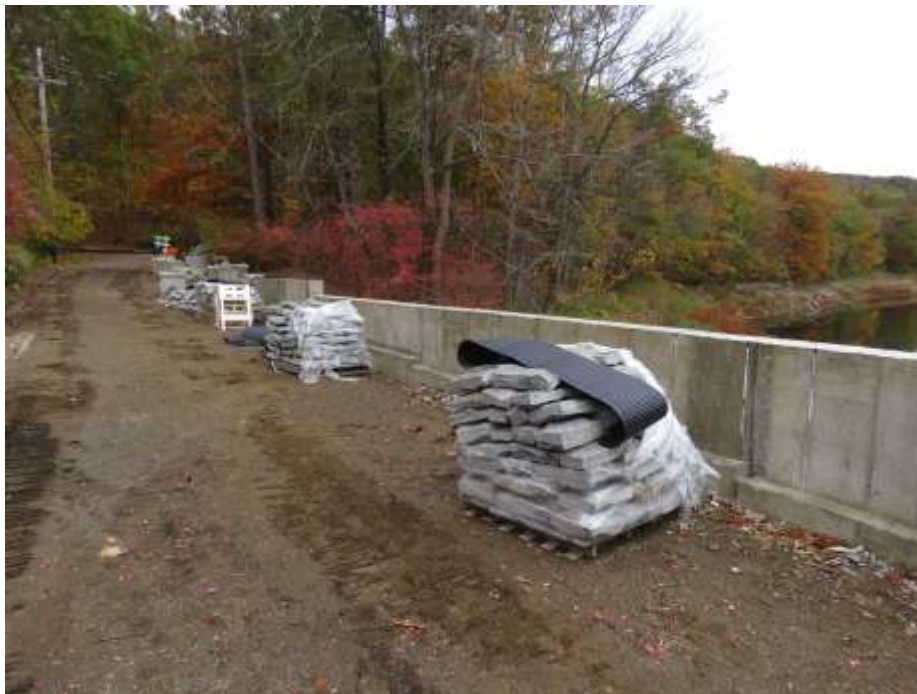
Completed reinforced concrete Segments E and D of Parapet Wall ready for stone effacement construction
