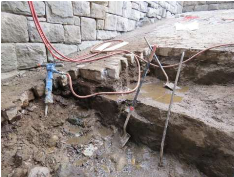
Excavation for repair auxiliary spillway floor.
