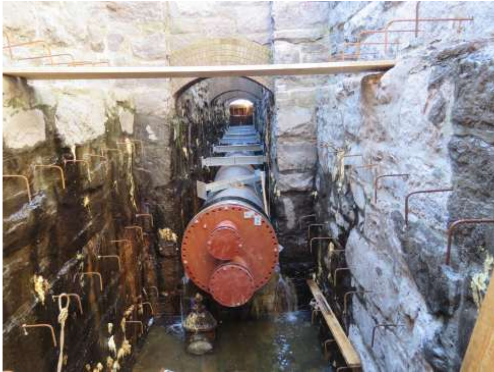
New low level outlet pipe set and braced in service spillway.
