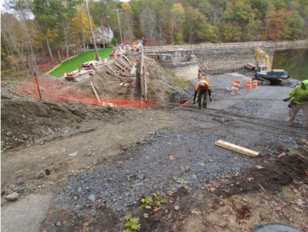
Reinforced concrete construction for Segment B of Parapet Wall.
