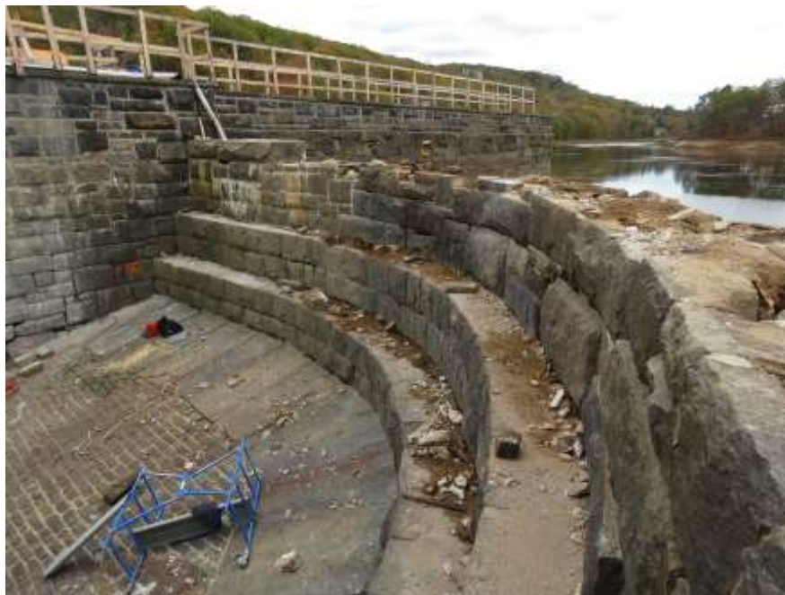
Capstone removal in preparation of auxiliary spillway crest reconstruction.
