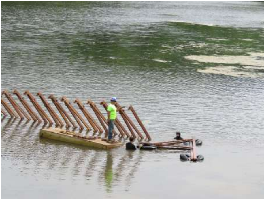
Contractor Assembling Temporary Cofferdam from Service Spillway to Left Abutment.
