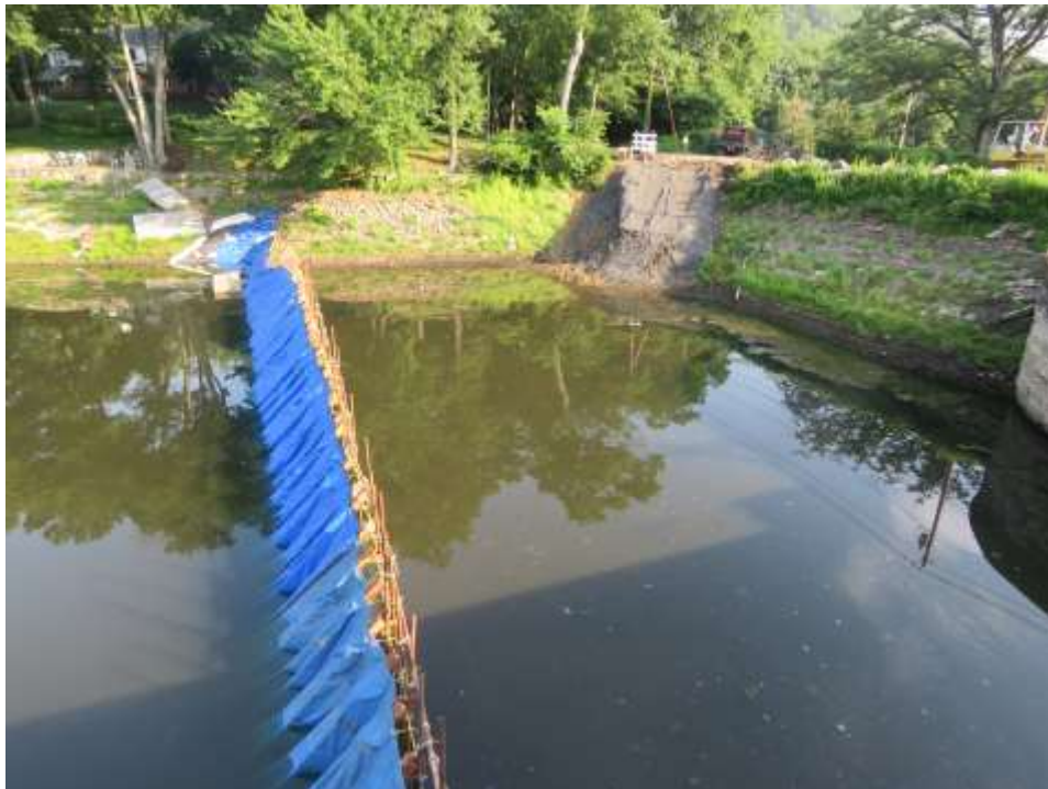
Completed Temporary Cofferdam and start of Dewatering of Coffered Area.
