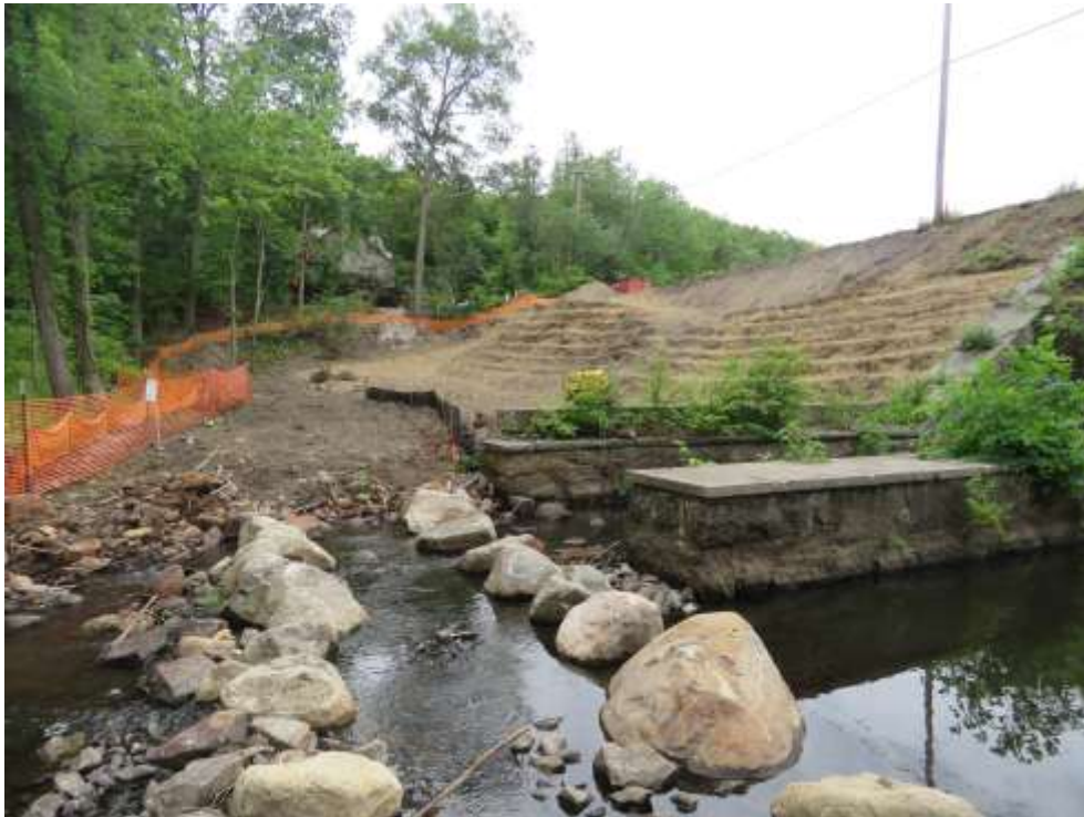
Right Side of Downstream Embankment Slope Following Clearing, Grubbing and Benching.
