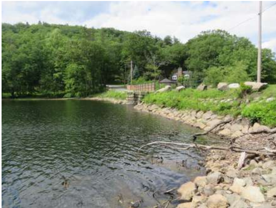
View of Pond No. 3 at Construction Pool. Dam Repairs and Modification Anticipated for Late Summer.
