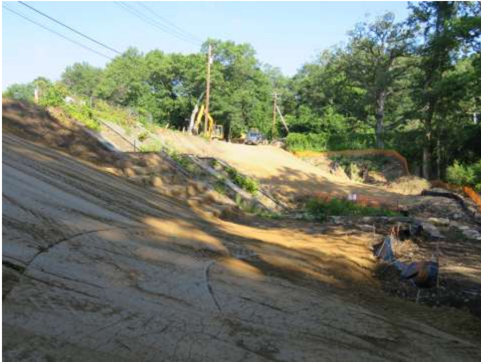
Compacted Embankment Filled on right Downstream Slope after Sealing with Compactor ahead of rain.
