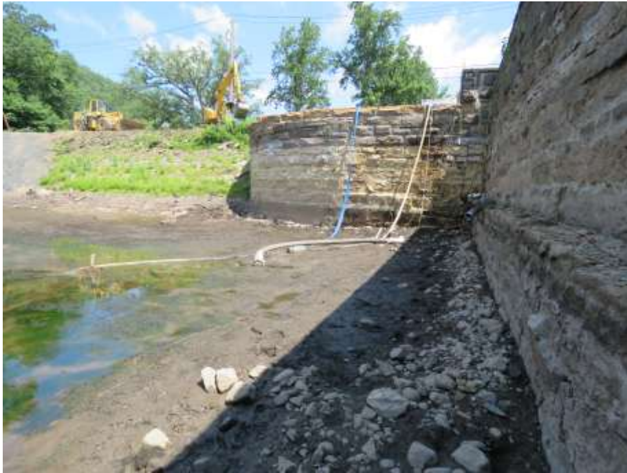
Dewatered Coffers Area Upstream of Auxiliary Spillway.
