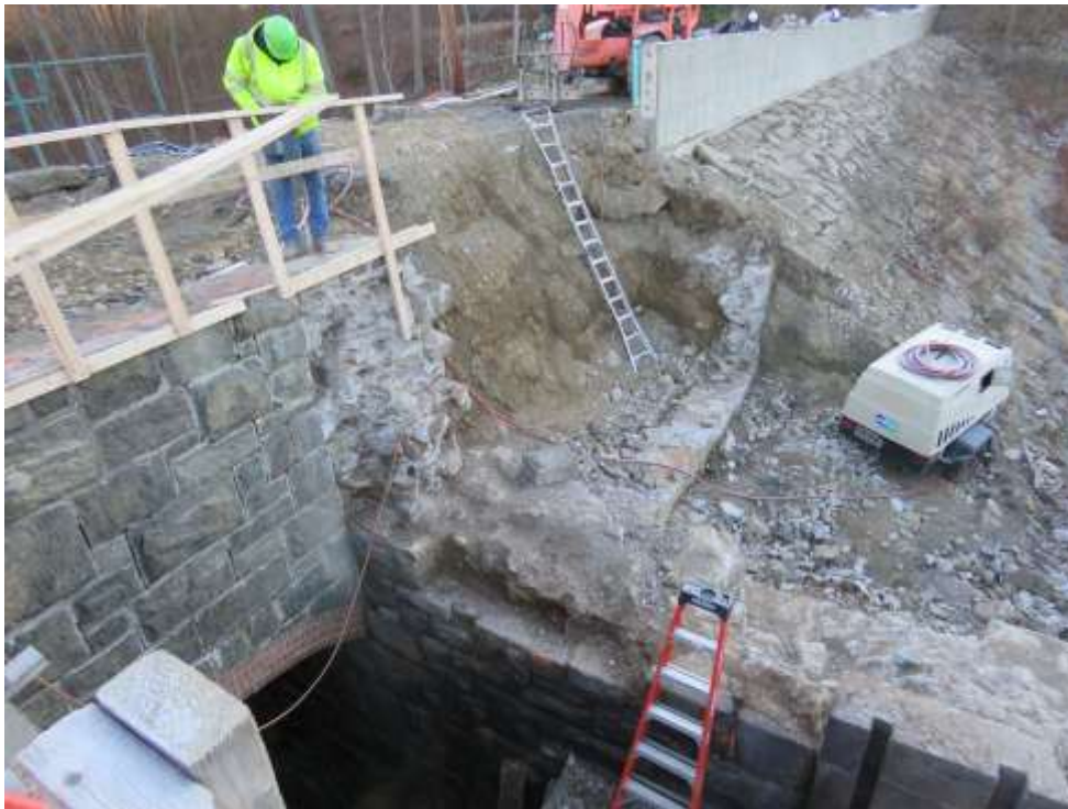
Forebay excavation and exposure of stone masonry cutoff wall (right side) within dam embankment.
