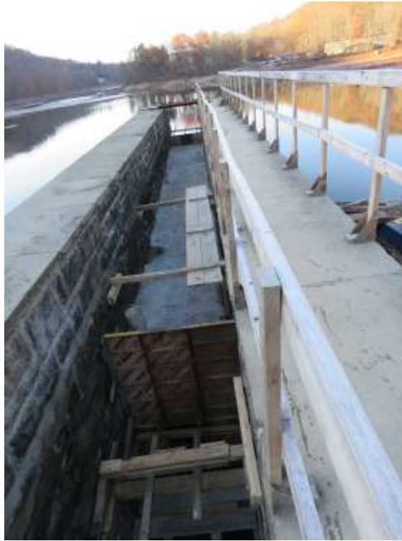
Service Spillway backfilled with mass concrete to elevation 491 ft.
