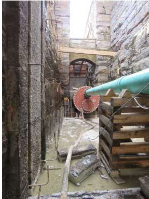
Construction of LLO within Service Spillway. Temporary PVC pipe used to convey base flow through construction area.
