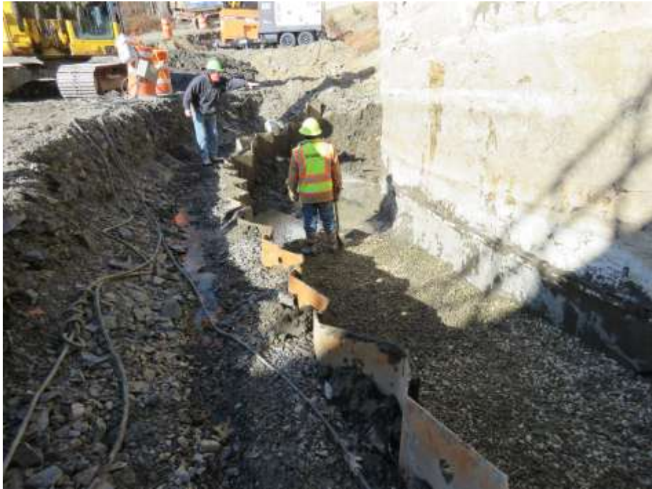
Sheet pile cutoff wall and excavation for auxiliary spillway overpour wall footing construction.
