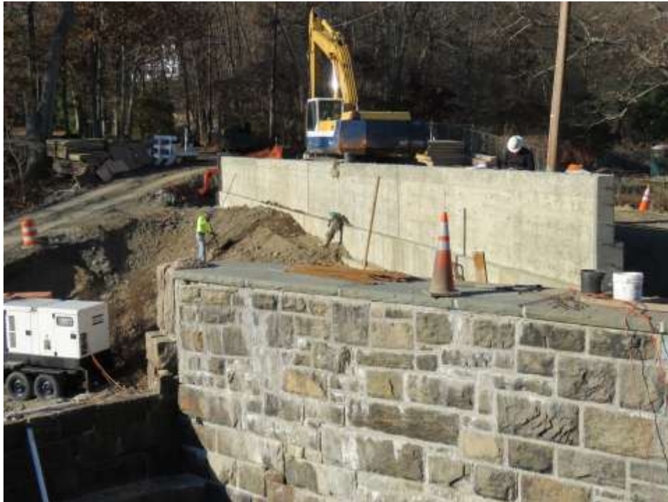
Construction of reinforced concrete parapet wall Segments B.
