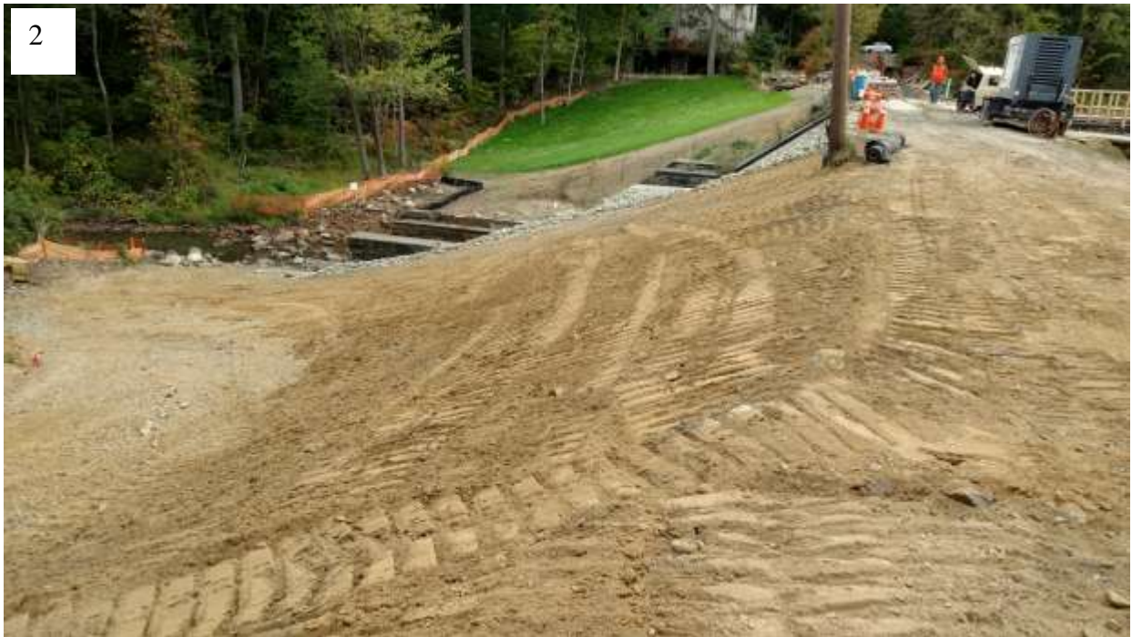
Completed left downstream slope grading prior to topsoil placement. Background shows completed embankment with temporary grass growth.
