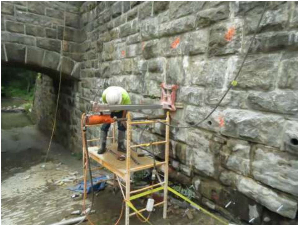
Coring operations in preparation of through bolt installations of the right auxiliary training wall.
