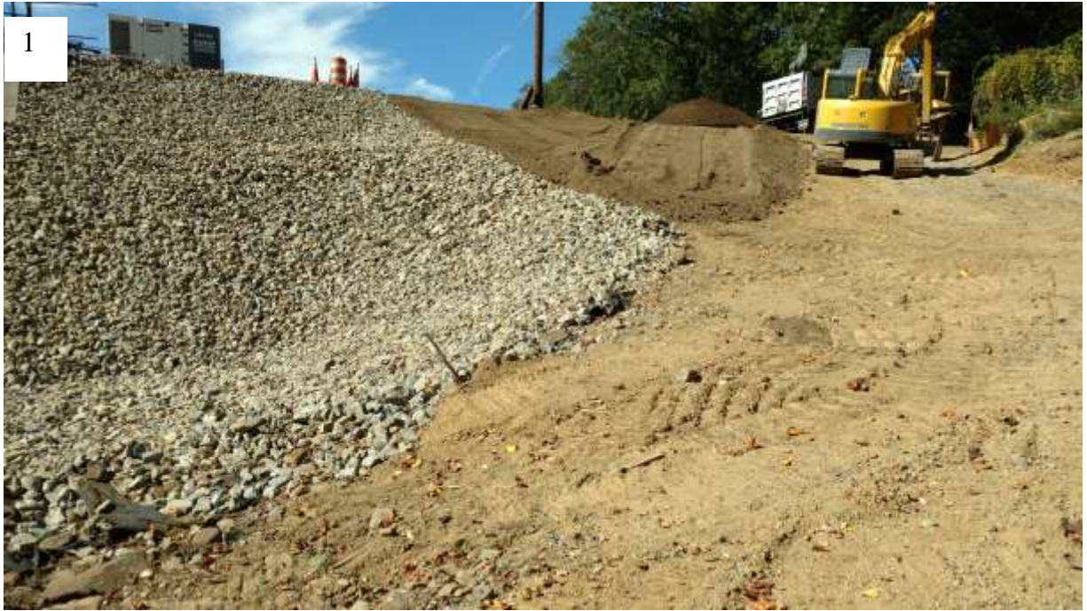
Left Side of Downstream Embankment Slope with Topsoil being place adjacent to rip rap slope protection placed to edge of service spillway discharge channel.
