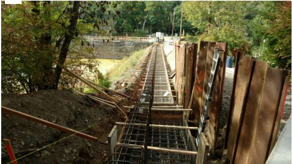
View of parapet wall segments E and D from right abutment of the dam just prior to concrete placement for base construction.
