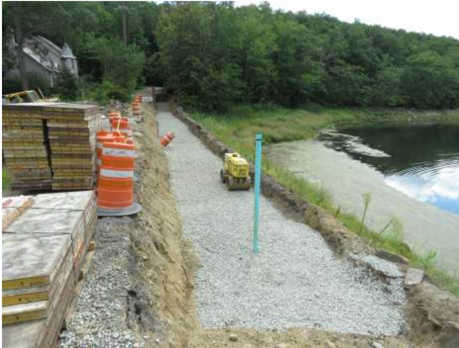
Parapet wall footing excavation. PVC pipe is casing of VW-Piezometer EM-5.
