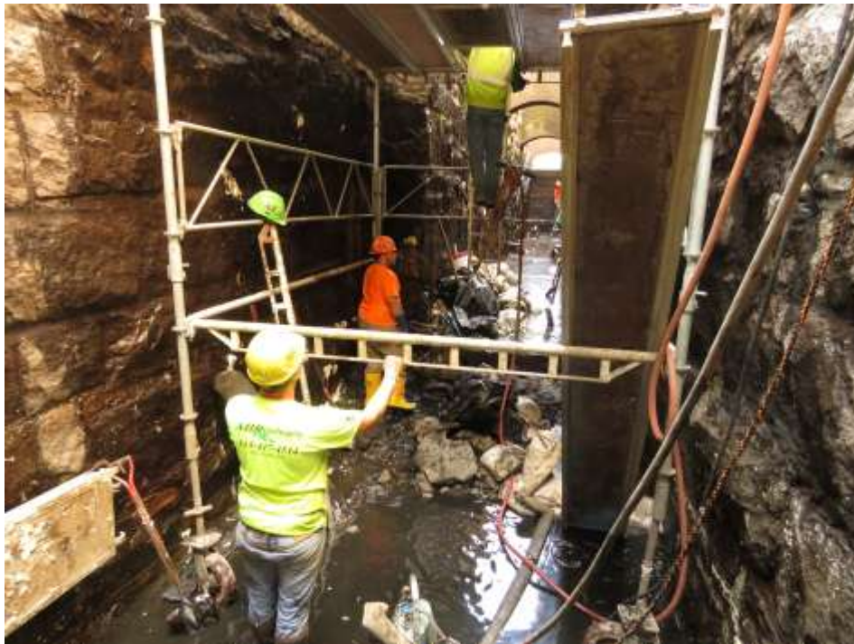
Debris Removal of Service Spillway Sump and 5.5' wide channel.
