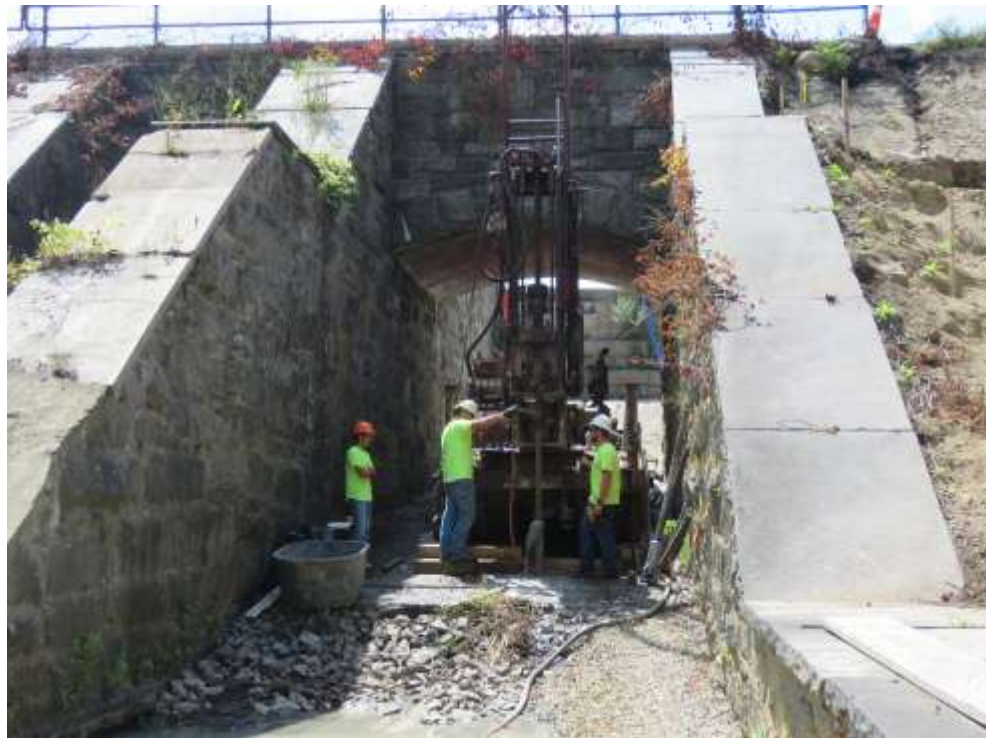
Looking Upstream in Auxiliary Spillway at drilling operations for VW-Piezometer Installation.
