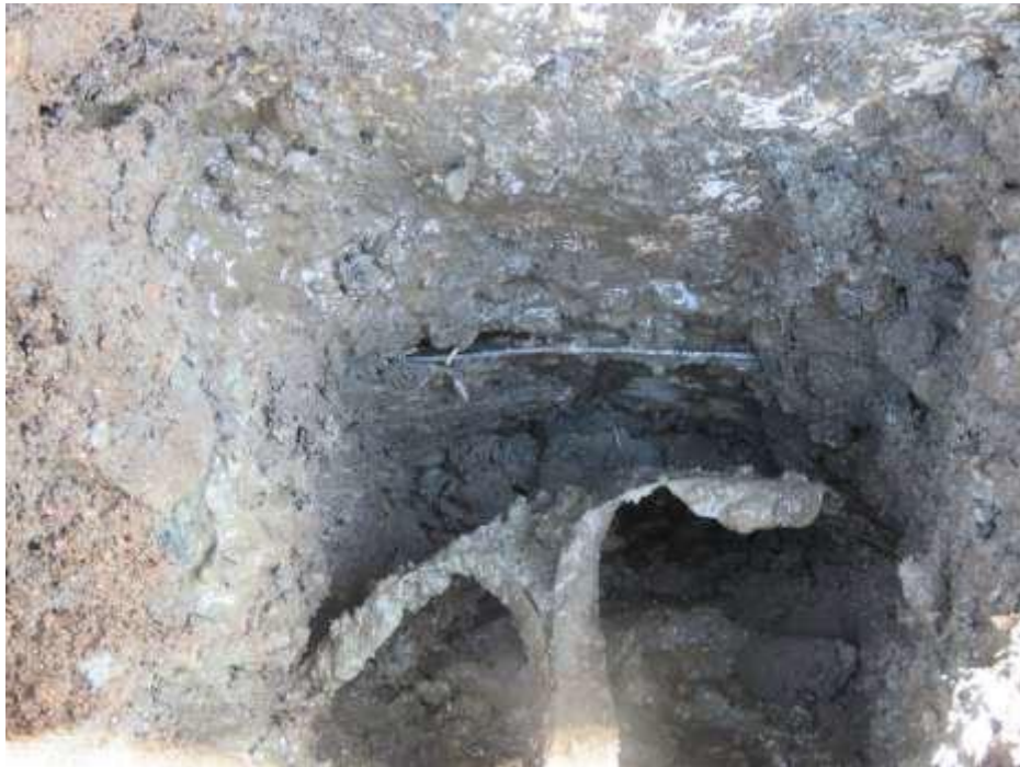
Existing Geomembrane (60 mil) Seepage Barrier at base of Auxiliary Spillway.
