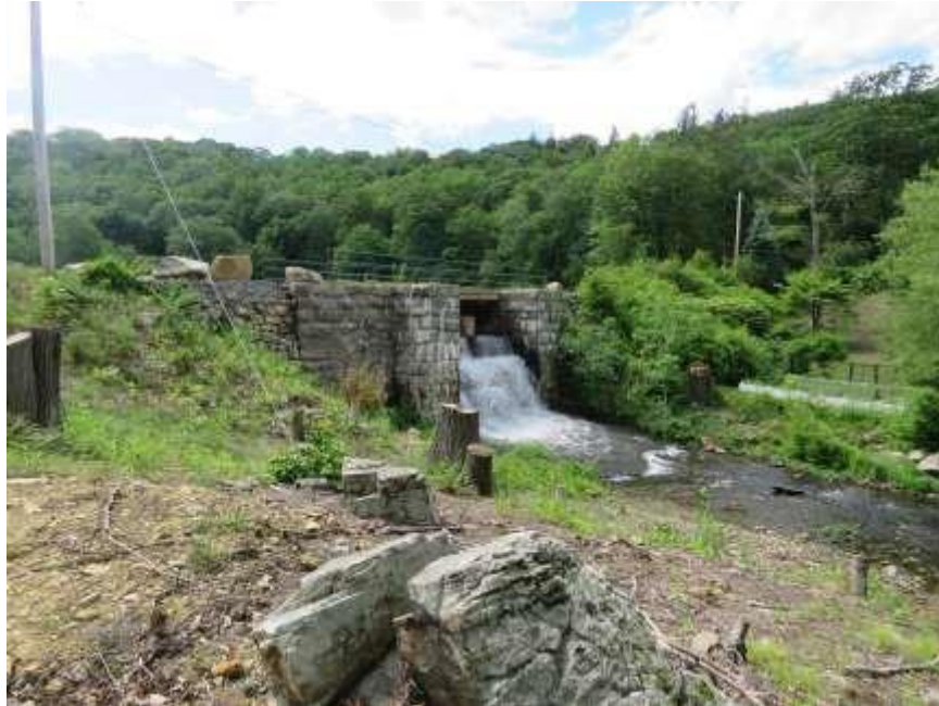
View of Pond No. 3 Dam Right Abutment/Embankment Contact and Primary Spillway.
