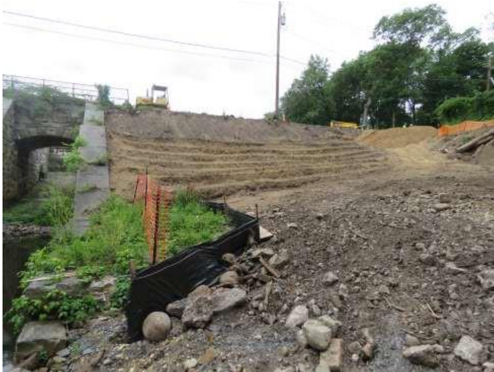
Left Side of Downstream Embankment Slope Following Clearing, Grubbing and Benching.
