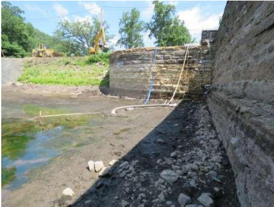
Dewatered Cofferd Area Upstream of Auxiliary Spillway.
