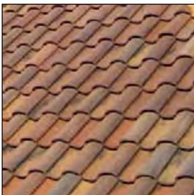
Replace damaged historic terra cotta roofing with new tiles that match original in material, color, decorative patterns and style.
