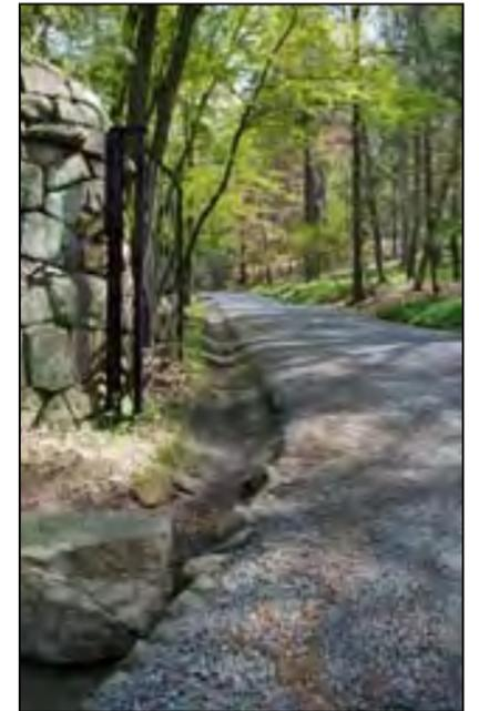
*Use natural materials for driveway surfaces and detailing. Provide rustic but effective and environmentally sustainable stormwater runoff measures.*
