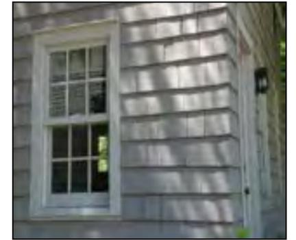
*Research original wood shingle type before starting a repair or restoration project. New shingles should be of high quality and replicate historic shingles in exposure and pattern.*
