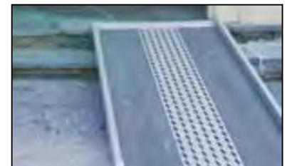
*Where possible, changes to historic entryways should be reversible. For example, a handicapped access ramp is installed in a manner that does not alter the original design of the steps and portico floor.*
