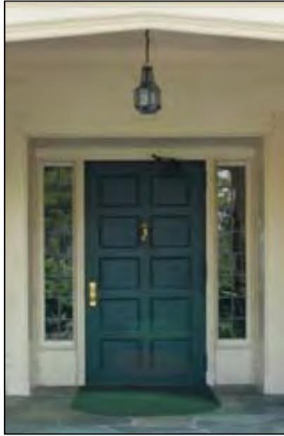
*Follow and adapt successful historic patterns. When repairing or replacing elements in the front entryway, match the original in sizes and scale. Retain as much original historic material as possible. Slope exterior surfaces away from the entry door. Only where deep shelter is provided can the entry material be flush with the door threshold, as in the example above.*
