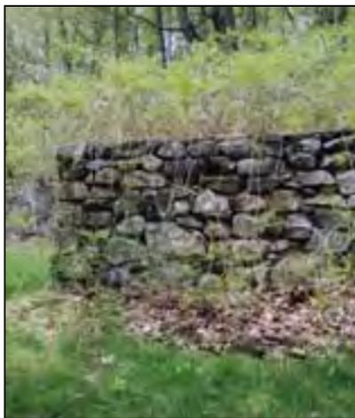
*New stone walls should replicate historic walls in stone placement and size. Local stone should be used.*
