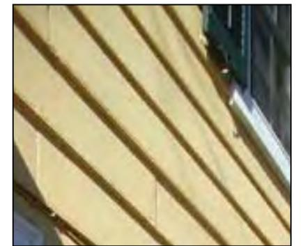
*Replicate original clapboard siding in exposure, detail and dimension. Install replacement clapboards of clear grade, solid material, and of a board length no less than 48 inches.*
