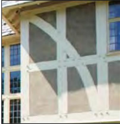
*Use brick masonry fill, nogging, wattle and daub, plaster or stucco fill with half timber construction. Non-traditional resin-based stuccos are not allowed for any repairs, restorations, additions or new construction.*
