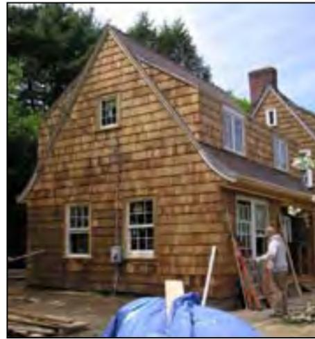
*Design additions that use building forms similar to those of the historic building. In this example, the roof shapes and lines of the original building are used on the addition. Also, the addition is lower in height and smaller in scale than the original.*
