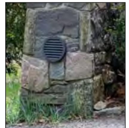
*An example of downlighting integrated into a stone gatepost.*
