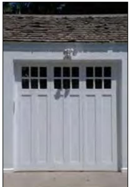
*Garage doors should be compatible with the character of the accessory building. Wood hinged doors are preferable. In cases where replacement is necessary, replace to imitate the original structure. Here the window size has changed, and the door is an overhead-swing model, while still matching the historic character.*
